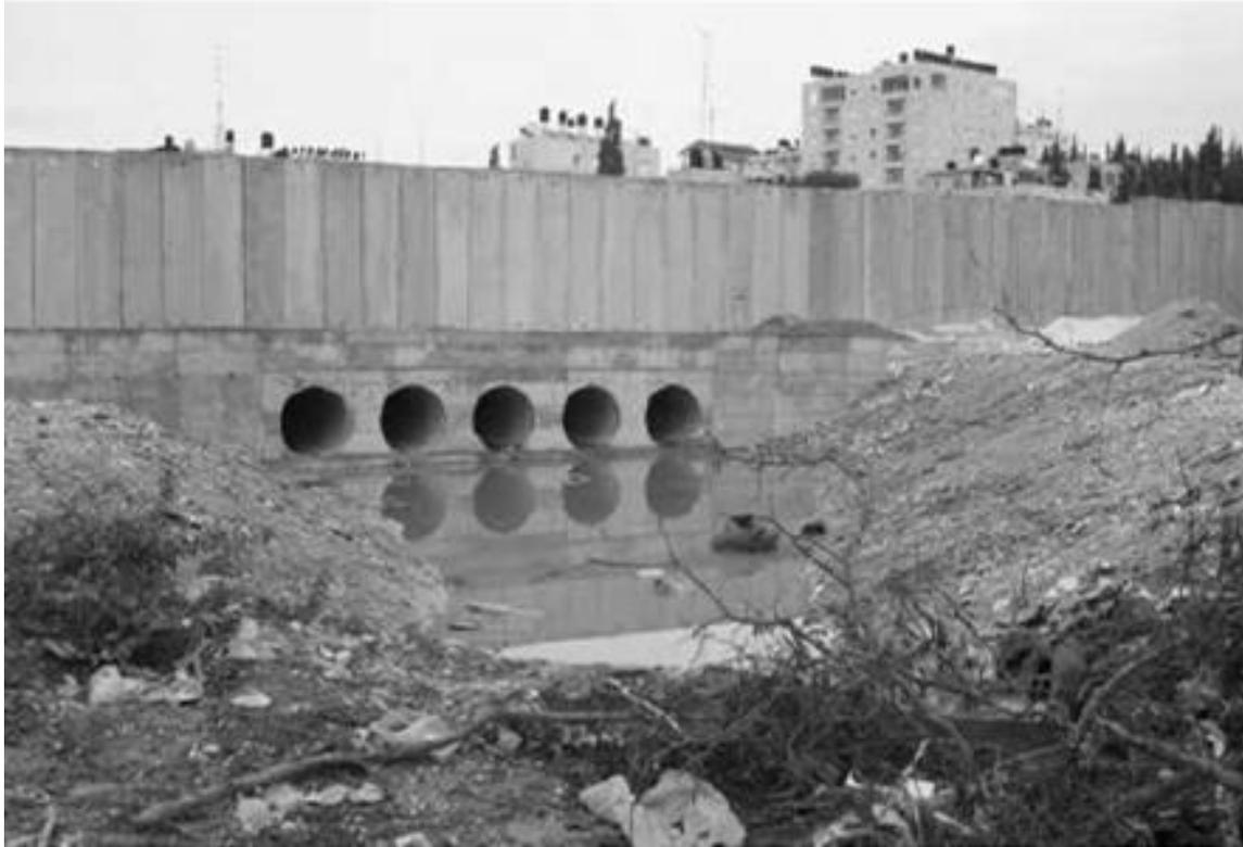
Figure 4-11 Sewage Overflow onto Open Lands due to the Cut of Sewage Network by the Separation Wall in Al Ram (after ARIJ, 2014)
