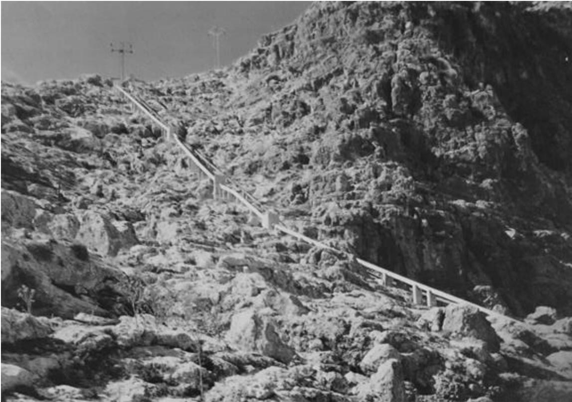
Figure 4-6 16" & 10" Conveying Lines between Main and Booster Stations Ein Samia (after JWU, 1995)
